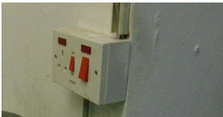
Cooker switch installed
